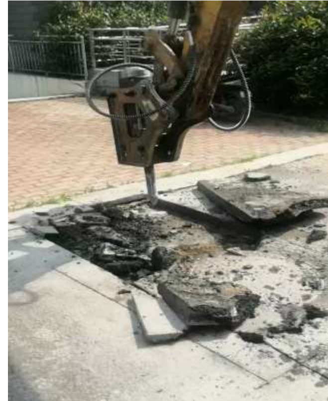
Pure hydraulic: Low impact force、Fast frequency、no need to press the drill rod
